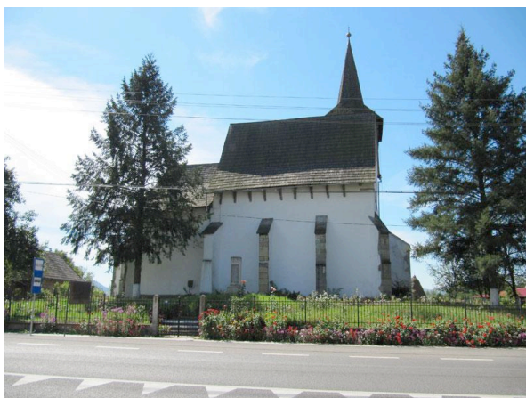
Fig. 6. The north side of the church and the buttresses.
