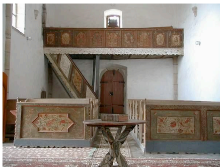
Fig. 9. The wooden ceiling of the space under the western gallery.
